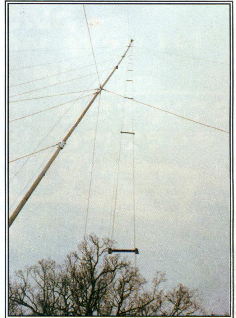
Open wire balanced twin feeder rising to the top of the mast
