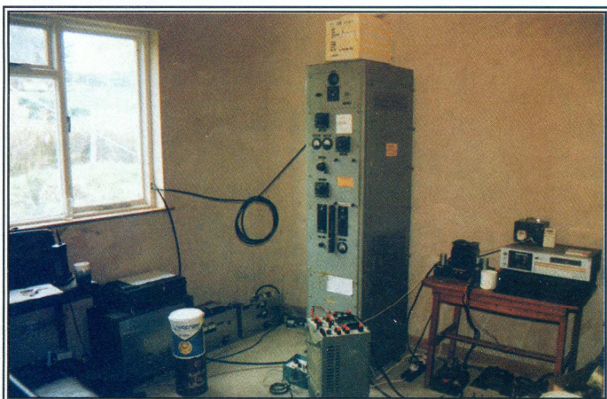
Engineering work in progress, Spring 1991
